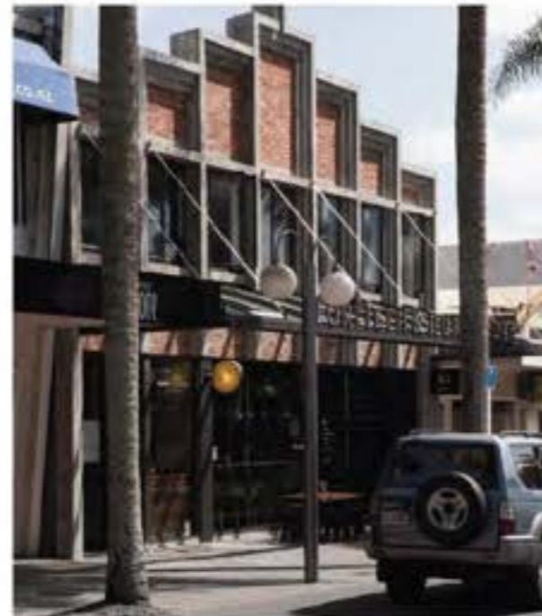
Fortleth and Hurstmere, Auckland Renovated character buildings to F&B
