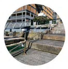
004. Existing handrail is easily climbable and allows jumping off the edge of the steps.
